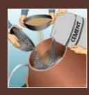
Charge cement and aggregates into the concrete mixer as per mix design Mix concrete mortar without adding water for 1-2 minutes
