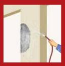
For priming of concrete substrate, the surface should be thoroughly saturated with potable water. Remove any excess of water prior to application
